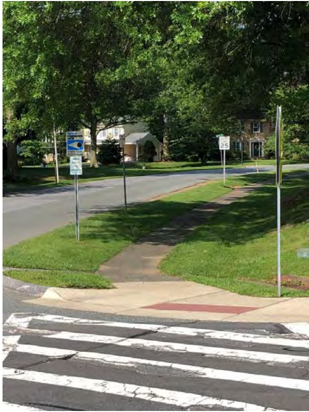
2. Narrow and poorly paved sidewalk on Cherry Valley Dr
