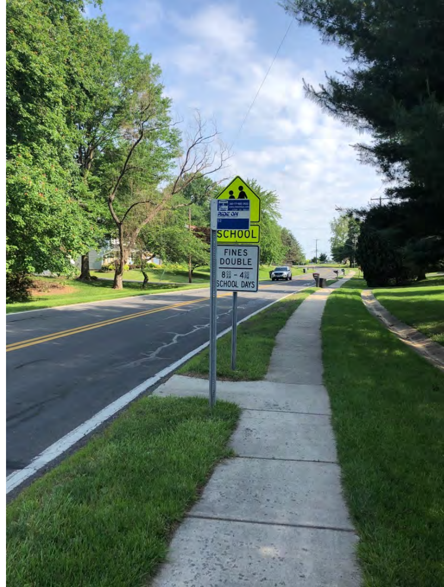
10. Ride On Bus sign blocks school zone signage.
