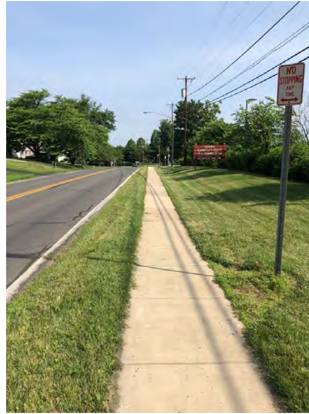
13. Narrow sidewalk along Cashell Rd
